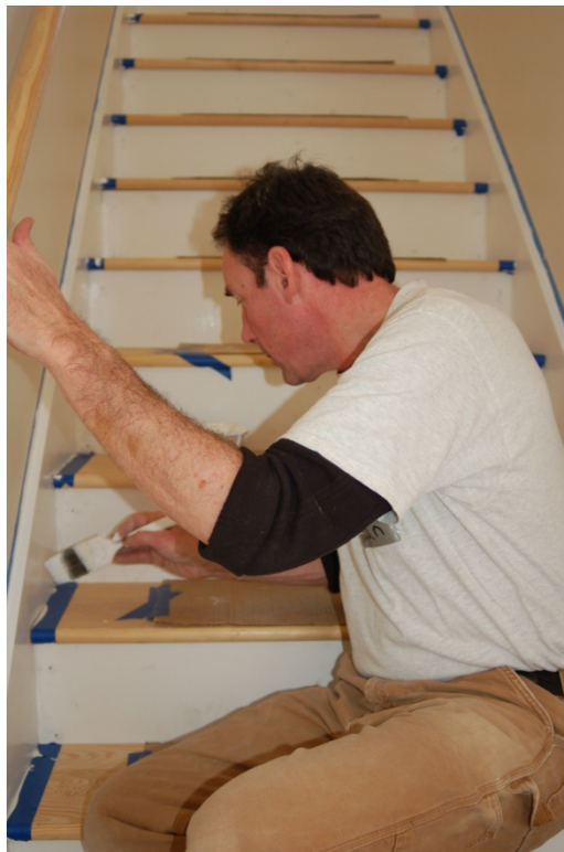
Sensei Dan Gobillot paints trim at the Habitat build site
